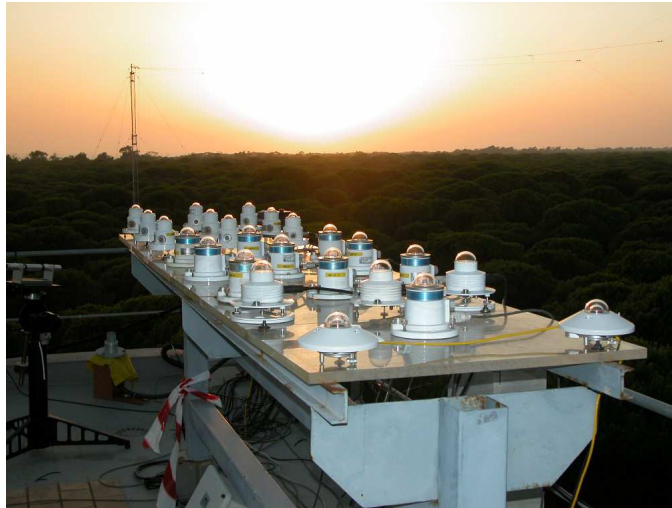
Figure 10: Broadband radiometers installed on the terrace of El Arenosillo Station.
